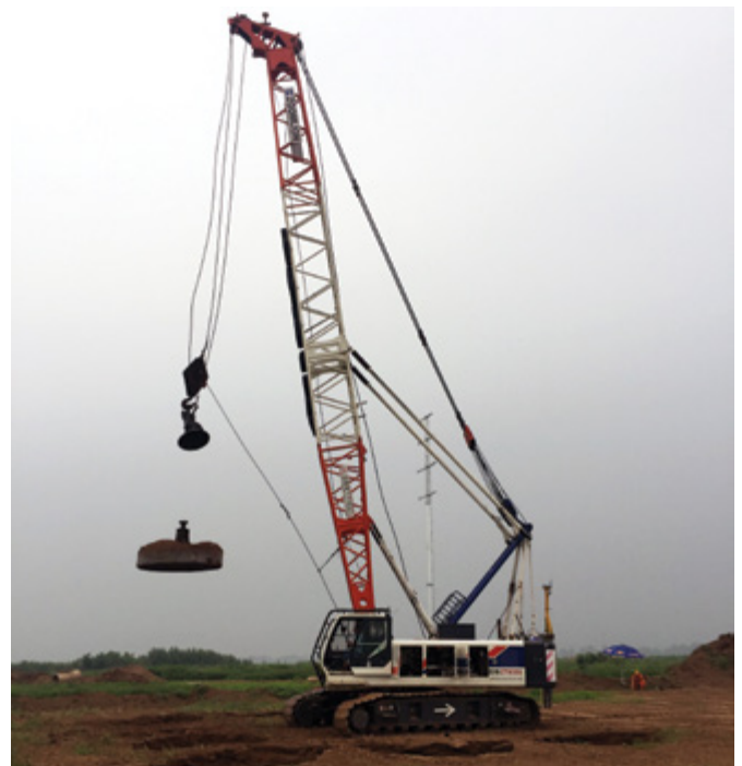
A crane was equipped with a GNSS-guided Trimble DPS900 Machine Control System to ensure maximum efficiency.
