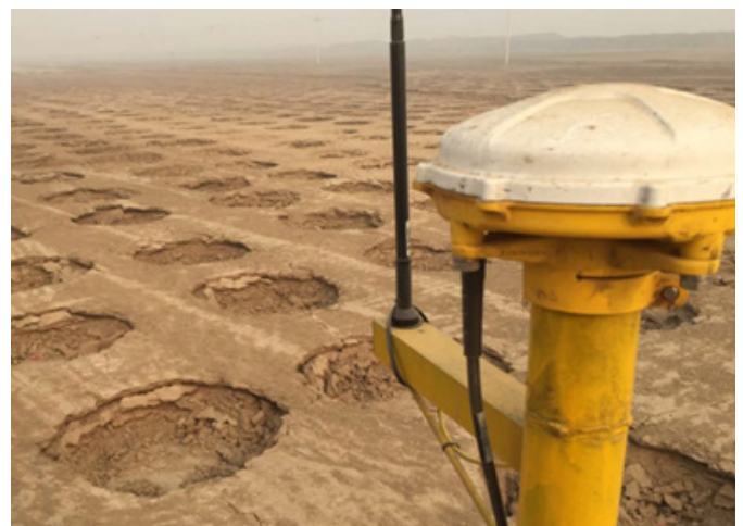
Accurate spacing between hammer drops was critical, but with a GNSS on-machine guidance system the compaction team easily achieved the accuracy they needed without stakes.
