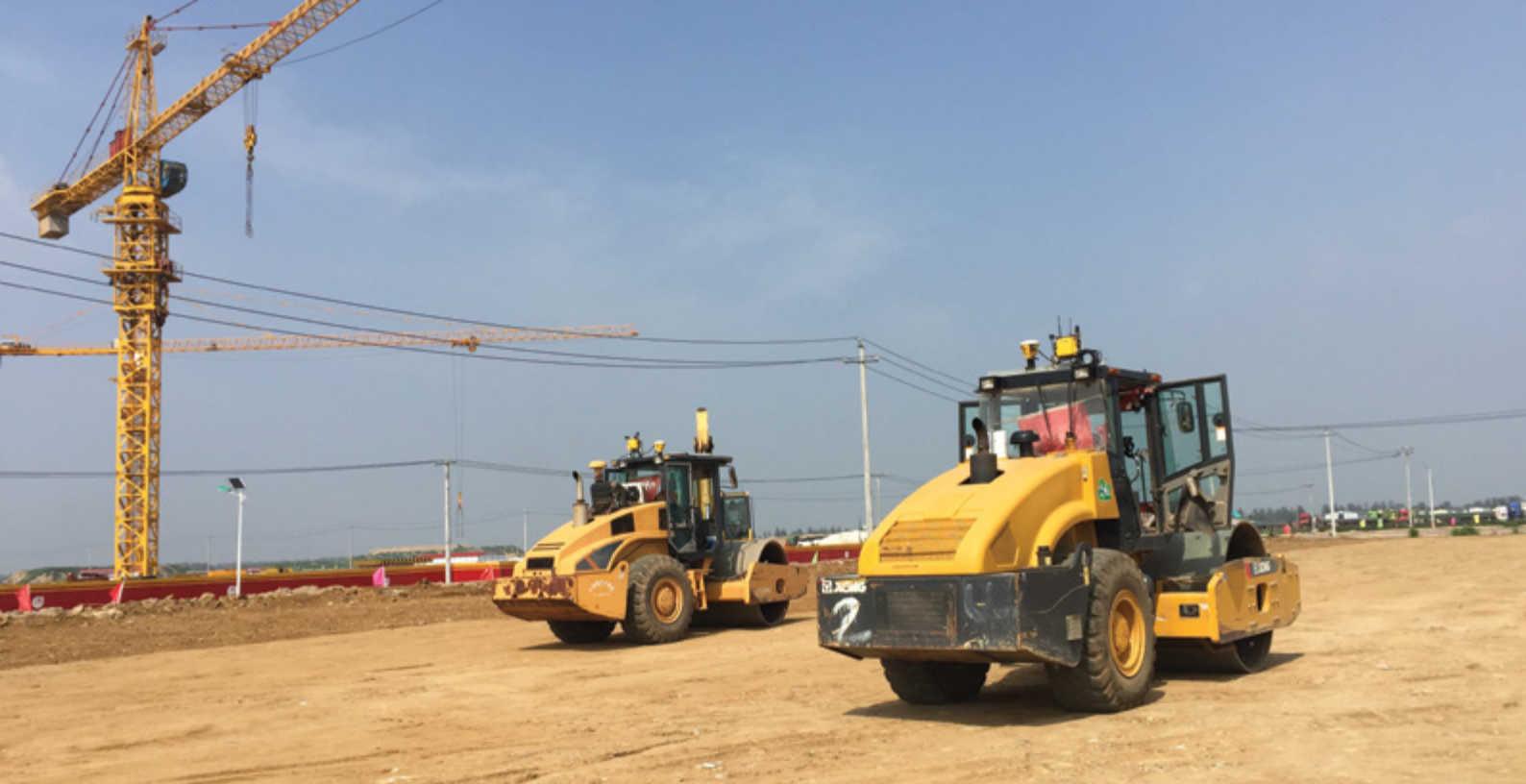
Other heavy machines for compaction were guided by the Trimble CCS900 Compaction Control System
