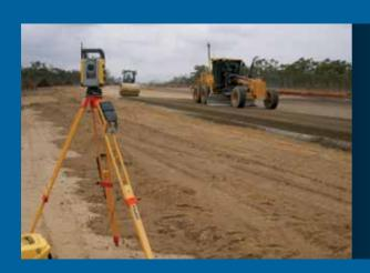
The grade control system accurately positions the blade in real time, improving the operators' productivity and profitability while minimizing material overages 9 9
